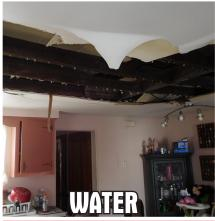
Flooding and water damage. Possible causes: Storms, bursting/leaking pipes, major drain clogs, faulty household appliances, leaking roof or windows, HVAC issues, improperly sloped landscaping.
