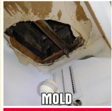
Mold growth in the house. Possible causes: cracked foundation, leaking pipes, damaged roof, poor ventilation, undetected water intrusion.
