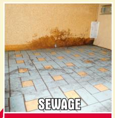
Sewage backup or leaks. Possible causes: Toilet clogs, main stack, floor drains, broken or leaking pipes.
