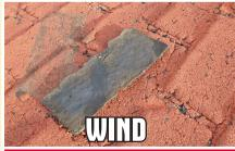
Exterior wind and weather damage. Possible causes: Existing problems with shingles and roof, airborne objects during a storm, loose siding and shutters, damaged flashing, hail and wind, improperly installed roof (i.e. valleys, flashing).
